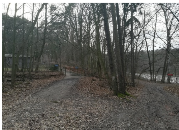
Fig. 5. Water treatment plant at Lake Kociołek (photo D. Węclewski)
